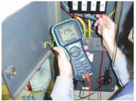
Checking the circuit continuity by multimeter
